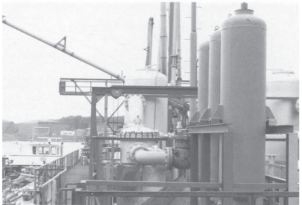
figure 1 HYDAC pulsation damper for reducing the pressure pulsations of 3 piston pumps, used in the pressure water supply station of a pickling plant.
